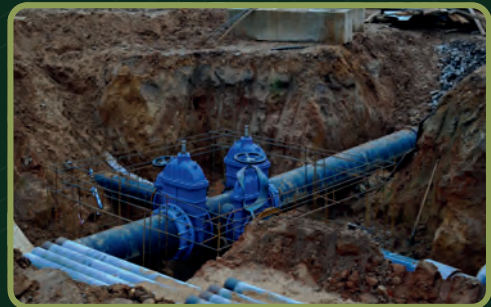
UNDERGROUND WATER PIPELINE
